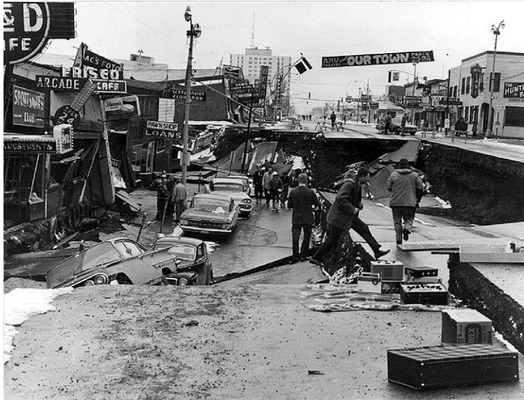
1964 Good Friday earthquake in Anchorage = magnitude 9.2, shook for nearly 5 minutes!
